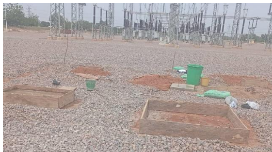
Figure 9: Clôture et fondation / Fence and foundations
