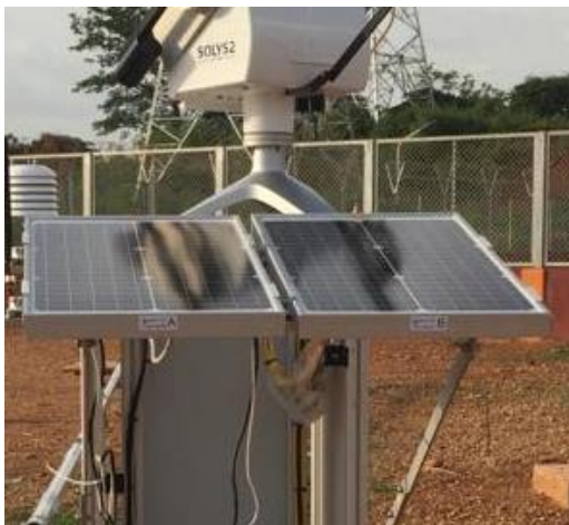
Figure 32: Assemblage de la structure PV-S + modules / Assembly of PV-S structure + modules.
