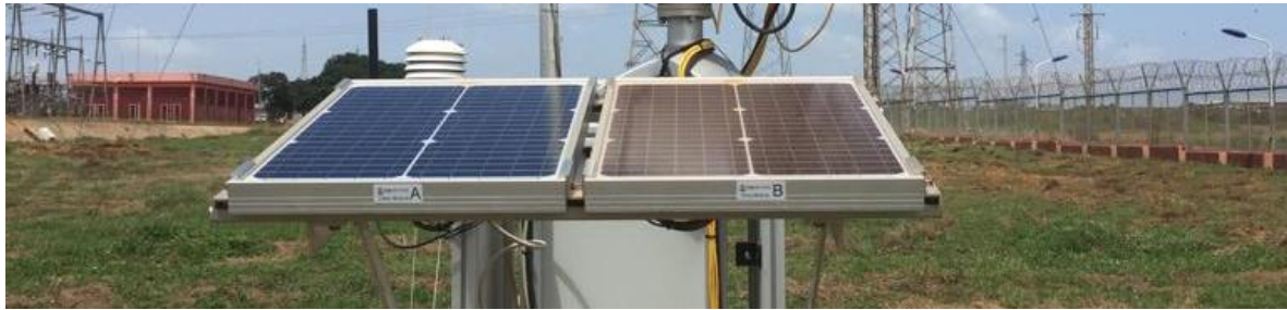
Figure 91: Assemblage de la structure PV-S + modules / Assembly of PV-S structure + modules.
