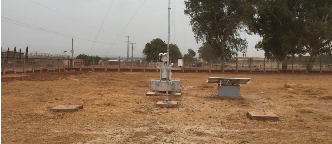
Figure 75 : Installation finale de la station vue du nord / Final station installation as seen from north.
