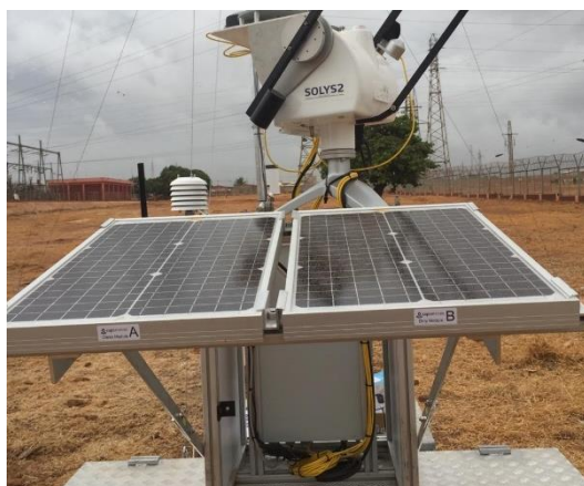
Figure 67: Assemblage de la structure PV-S + modules / Assembly of PV-S structure + modules.
