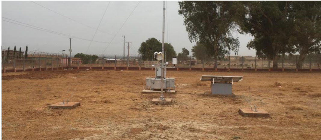
Figure 40 : Installation finale de la station vue du nord / Final station installation as seen from north
