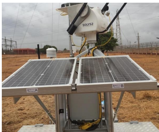
Figure 32: Assemblage de la structure PV-S + modules / Assembly of PV-S structure + modules.
