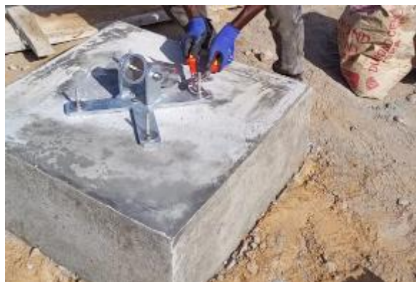
Figure 45: Fondations du mât du vent / Wind mast foundations.
