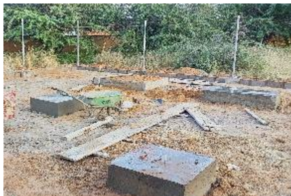
Figure 44: Clôture et fondation / Fence and foundations.
