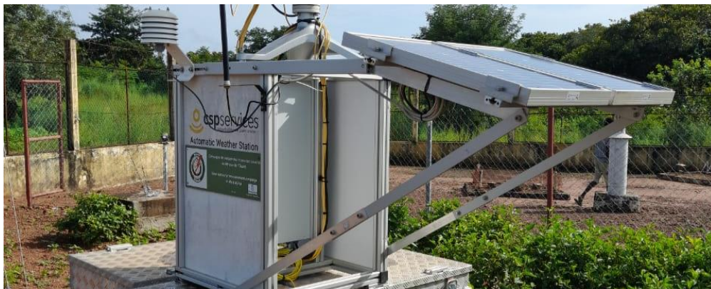
Figure 87: Assemblage de la structure PV-S + modules / Assembly of PV-S structure + modules.
