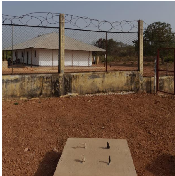
Figure 45: Fondations du mât du vent / Wind mast foundations.
