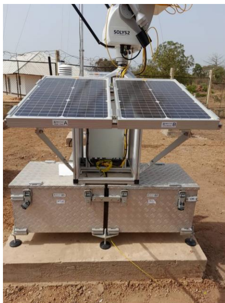
Figure 32: Assemblage de la structure PV-S + modules / Assembly of PV-S structure + modules.
