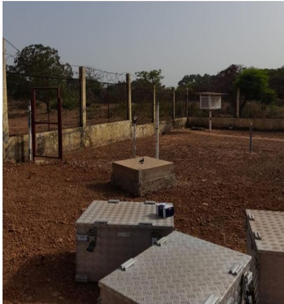
Figure 9: Clôture et fondation / Fence and foundations
