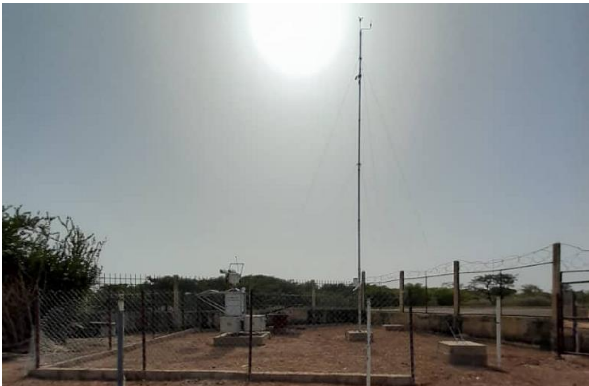
Figure 41 : Installation finale de la station vue de l'est / Final station installation as seen from east.
