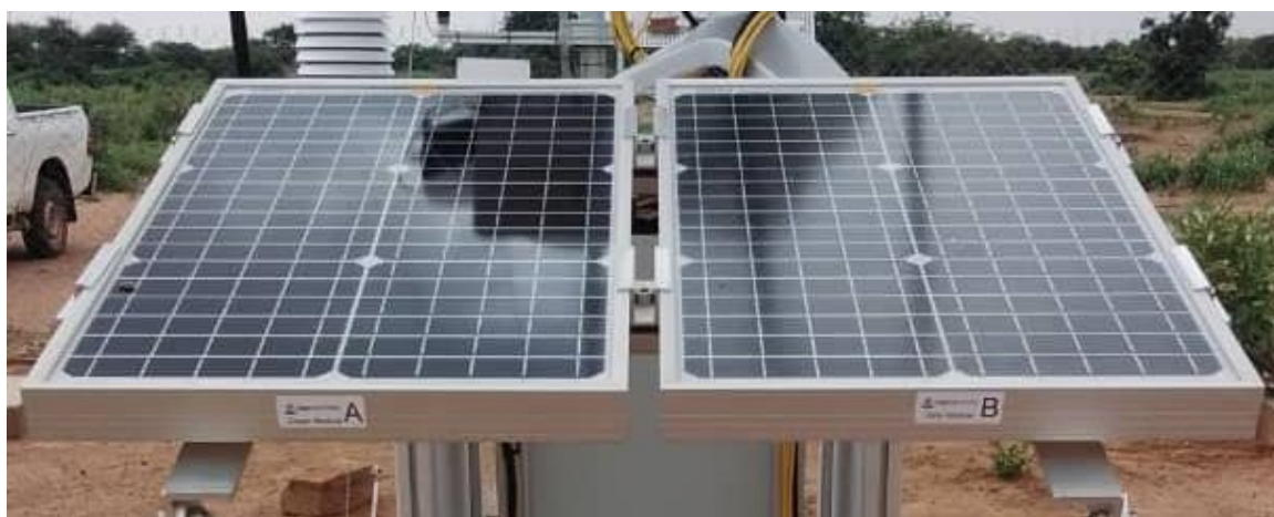
Figure 85: Assemblage de la structure PV-S + modules / Assembly of PV-S structure + modules.
