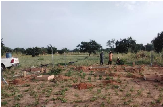
Figure 44: Clôture et fondation / Fence and foundations.
