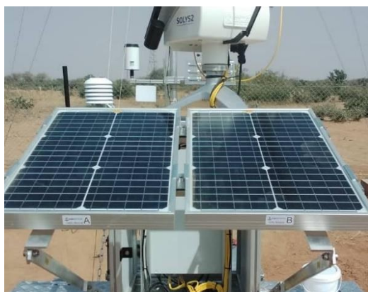
Figure 67: Assemblage de la structure PV-S + modules / Assembly of PV-S structure + modules.
