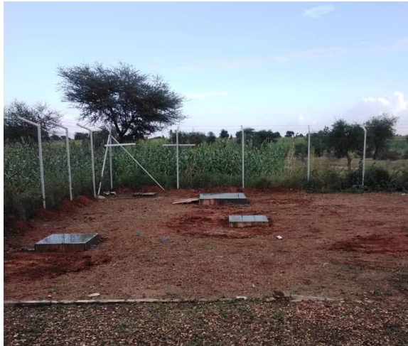
Figure 9: Clôture et fondation / Fence and foundations
