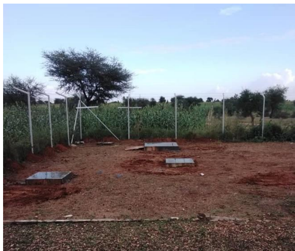
Figure 45: Clôture et fondation / Fence and foundations.
