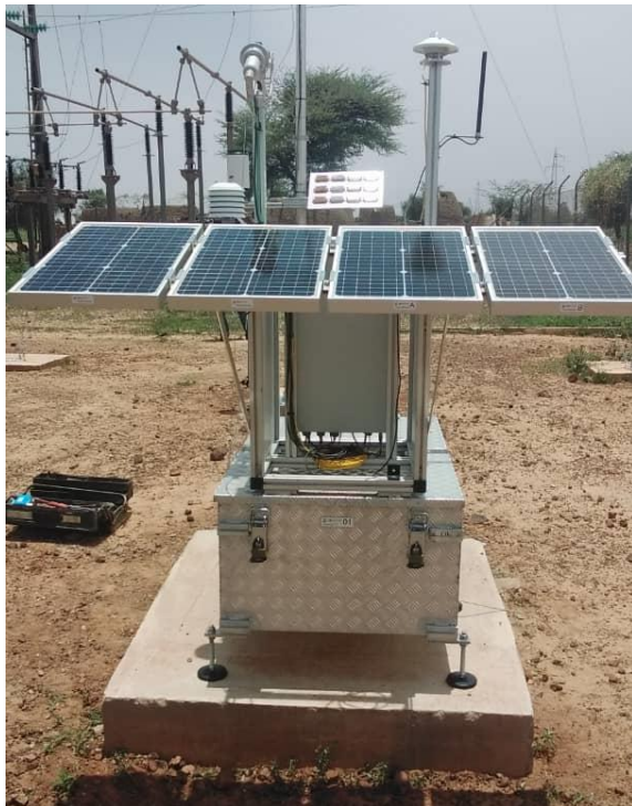
Figure 84: Assemblage de la structure PV-S + modules / Assembly of PV-S structure + modules.
