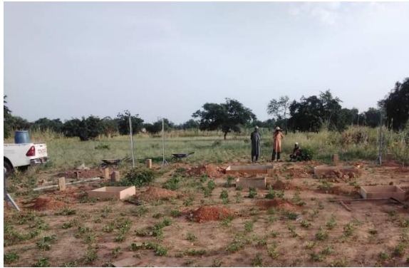
Figure 9: Clôture et fondation / Fence and foundations
