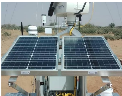
Figure 32: Assemblage de la structure PV-S + modules / Assembly of PV-S structure + modules.
