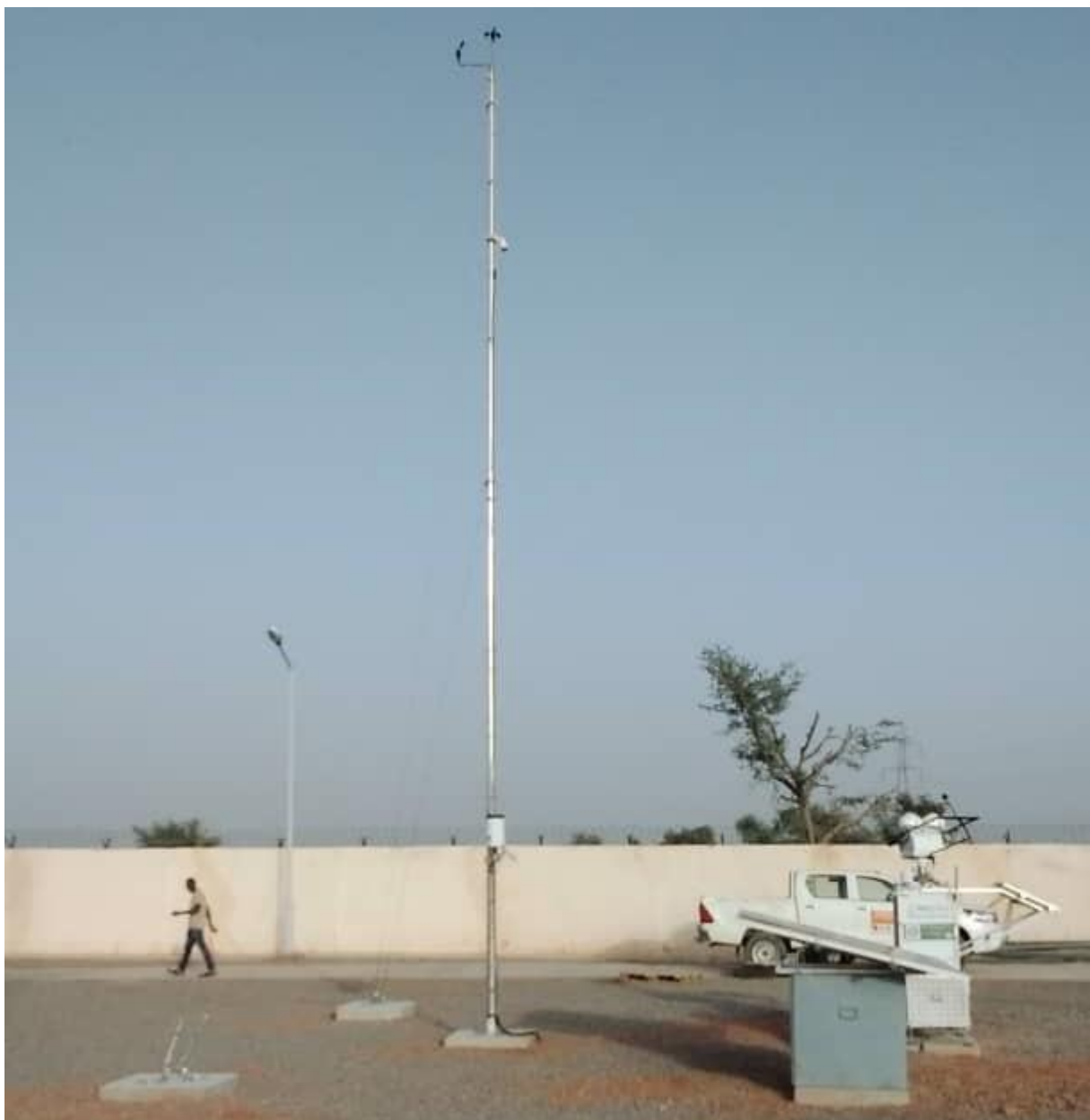
Figure 76 : Installation finale de la station vue du ouest / Final station installation as seen from west.
