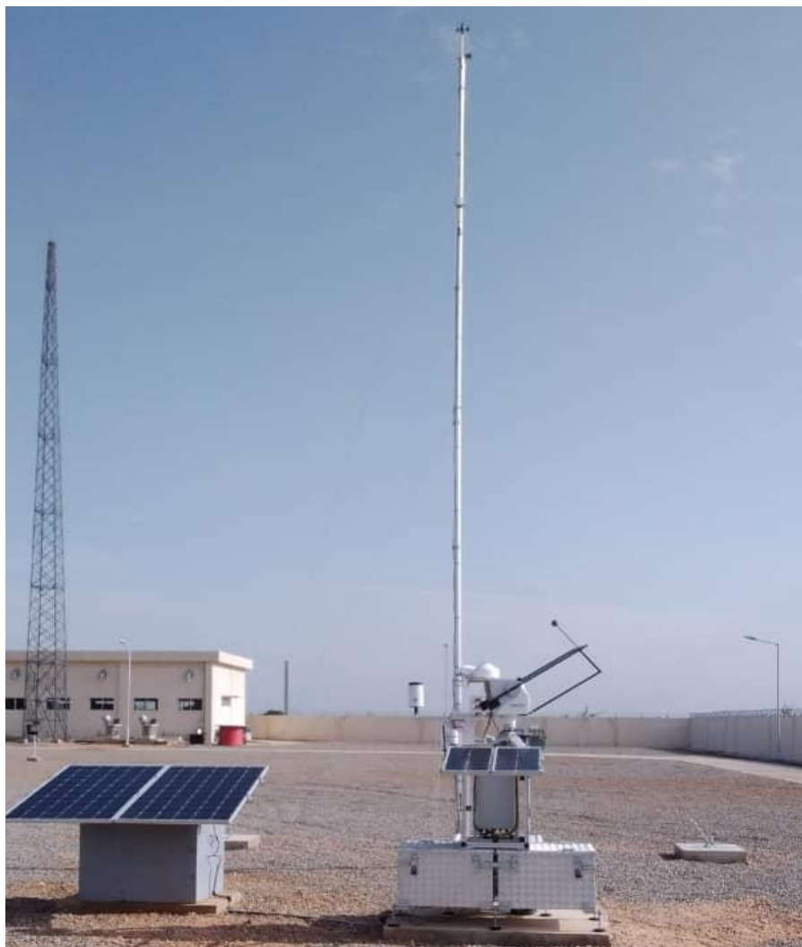
Figure 93 : Vue générale de la station / General view of the station.
