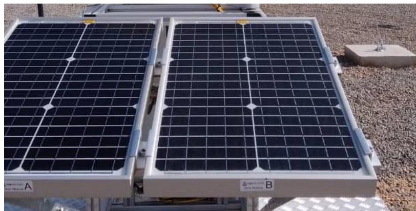
Figure 87: Assemblage de la structure PV-S + modules / Assembly of PV-S structure + modules.
