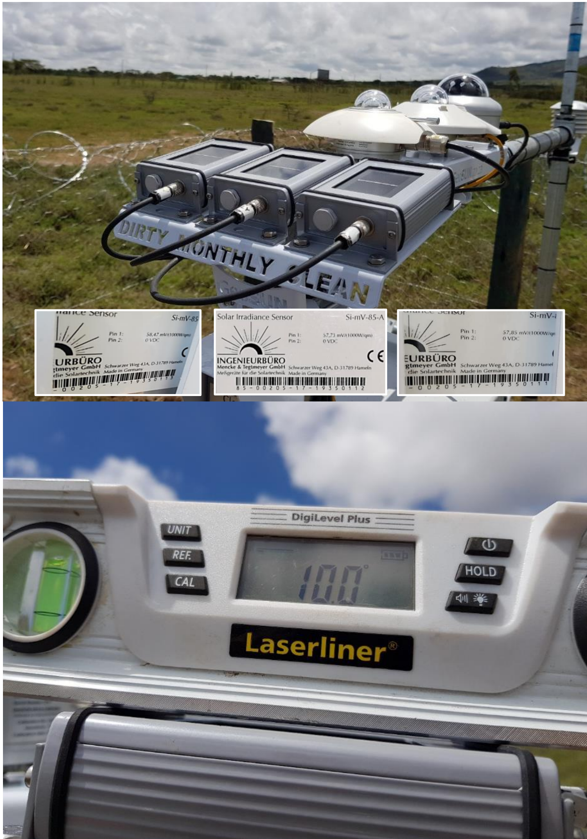
Figure 15: Reference Cells at 10° North
