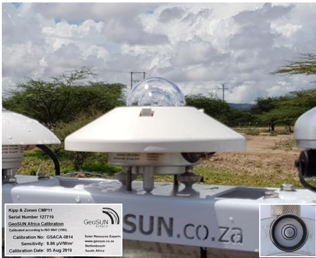
Figure 8: GHI (2) Pyranometer Installation
