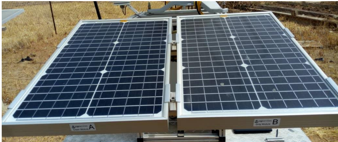
Figure 86: Assemblage de la structure PV-S + modules / Assembly of PV-S structure + modules.
