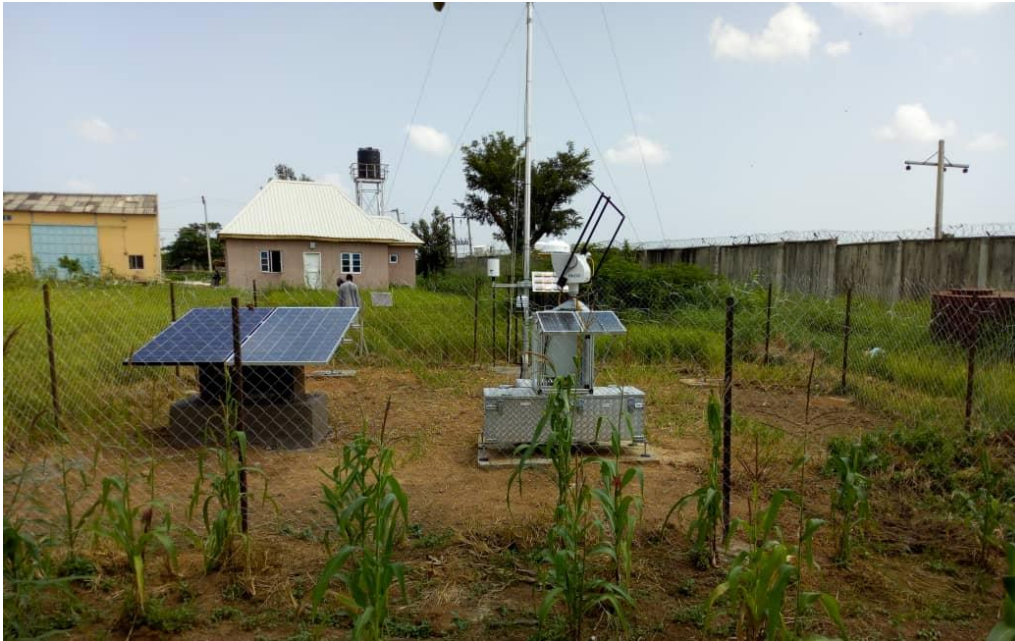
Figure 74 : Installation finale de la station vue du sud / Final station installation as seen from south.
