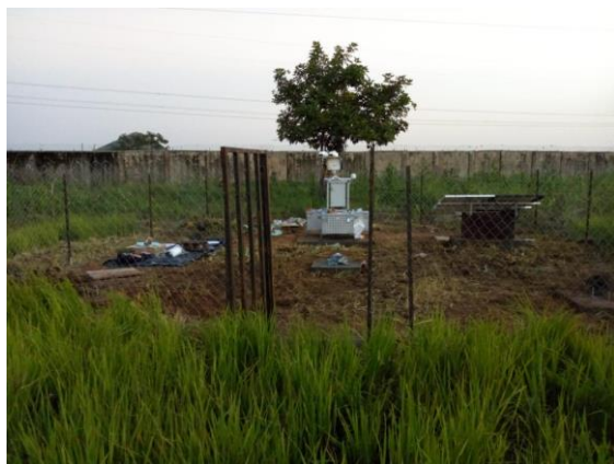
Figure 44: Clôture et fondation / Fence and foundation.
