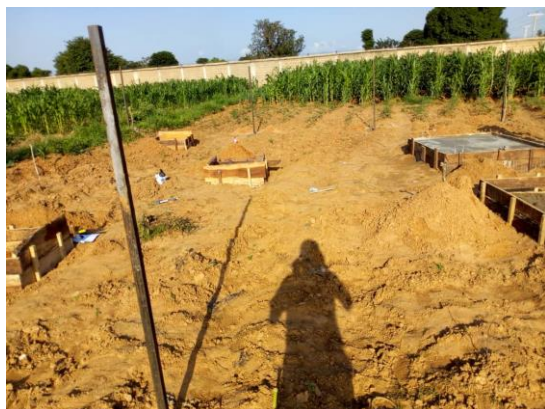
Figure 44: Clôture et fondation / Fence and foundation.
