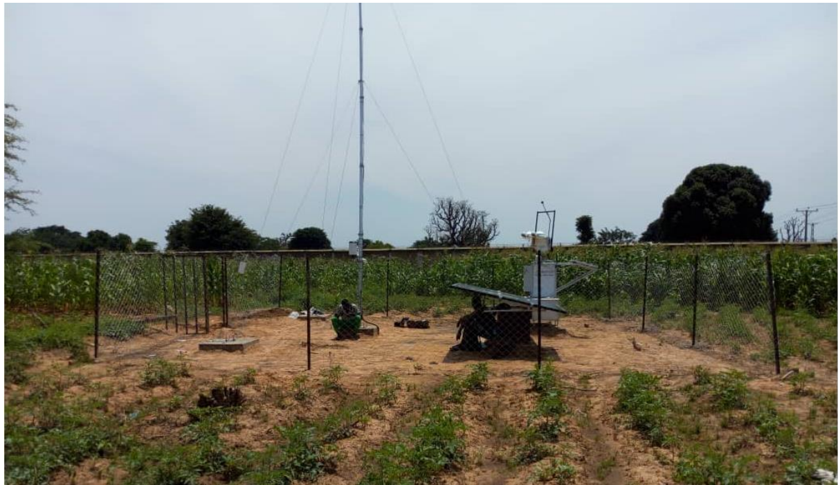
Figure 74 : Installation finale de la station vue de l'ouest / Final station installation as seen from west.
