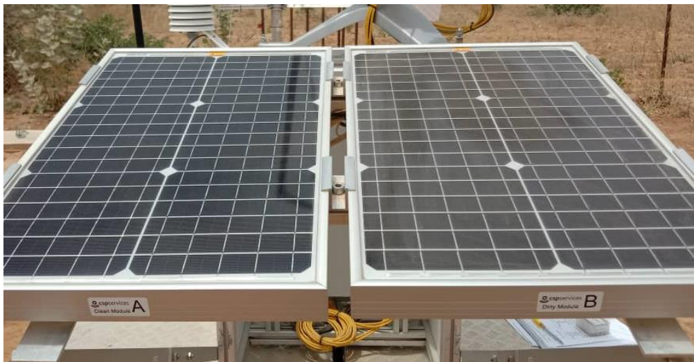
Figure 90: Assemblage de la structure PV-S + modules / Assembly of PV-S structure + modules.
