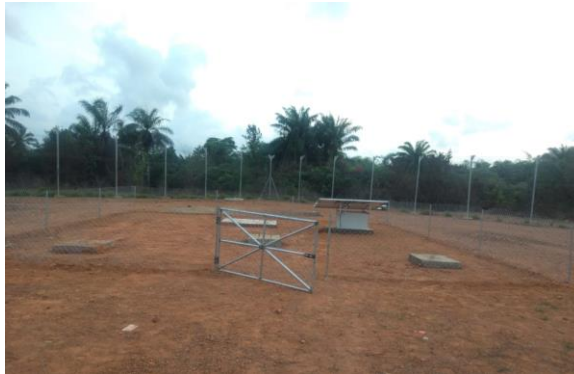
Figure 9: Clôture et fondation / Fence and foundations
