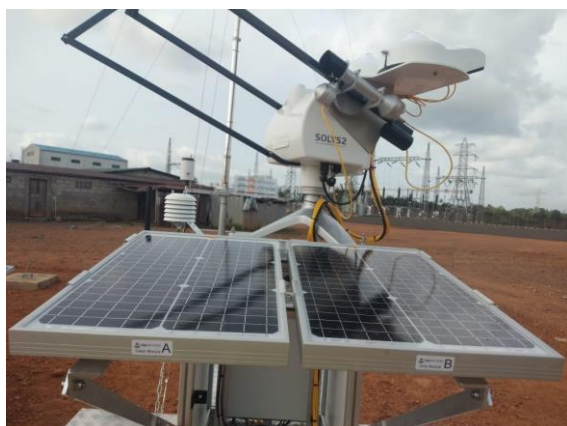
Figure 32: Assemblage de la structure PV-S + modules / Assembly of PV-S structure + modules.
