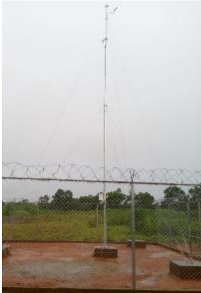
Figure 17 - Wind mast erected; wind direction sensor cantilever orientated to North
