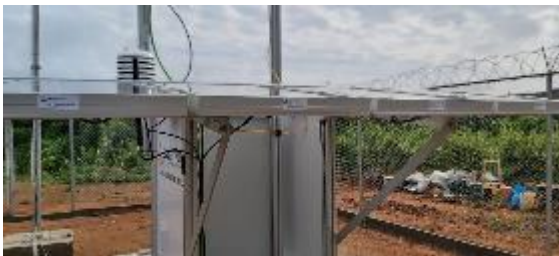
Figure 33 - Assembly of PV-S structure + modules
