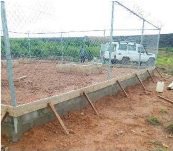
Figure 9 - Fence and foundation
