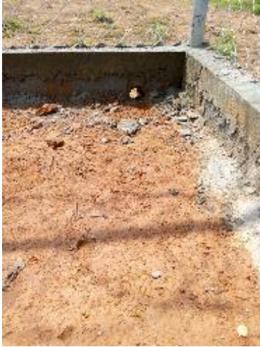
Figure 13 - Water holes in foundations to prevent flooding (1).
