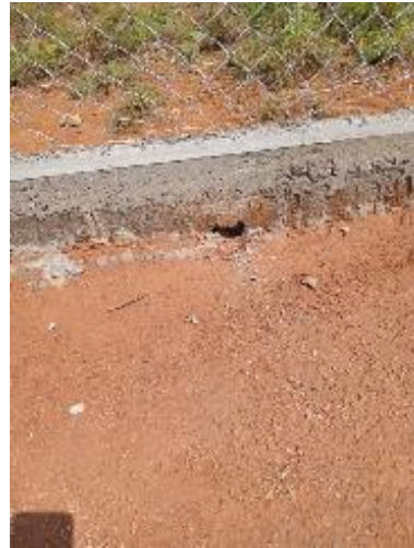
Figure 14 - Water holes in foundations to prevent flooding (2).
