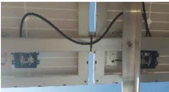
Figure 35 - PV-S modules connections
