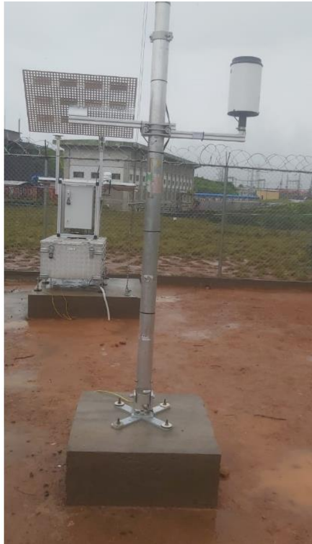
Figure 39 - Wind mast with rain sensor and corrosion sampler
