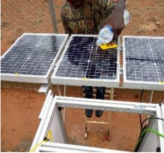
Figure 37 - PV modules cleaning.
