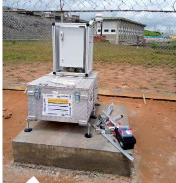
Figure 18 - Mounting of weather station structure
