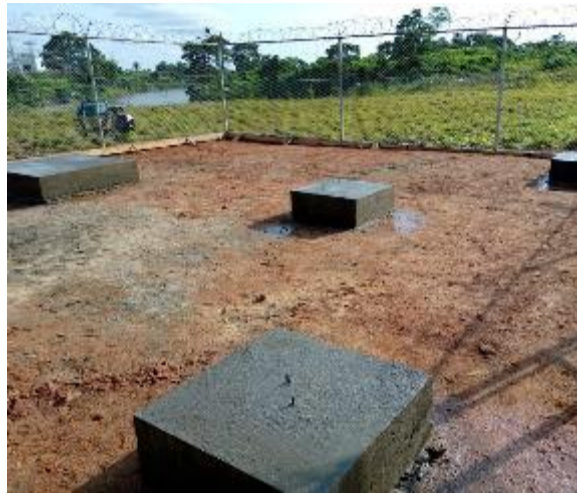
Figure 10 - Station and wind mast foundations
