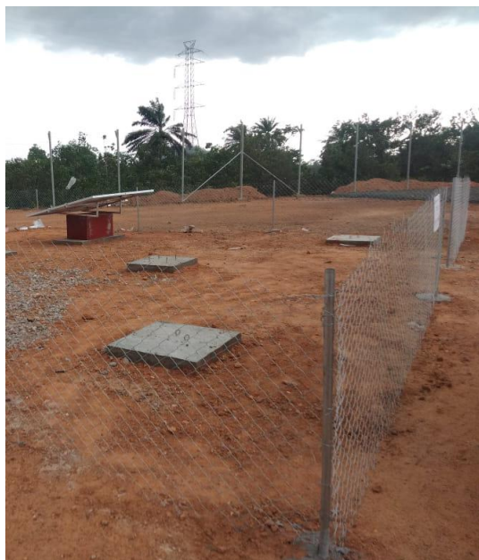
Figure 44: Clôture et fondation / Fence and foundations.
