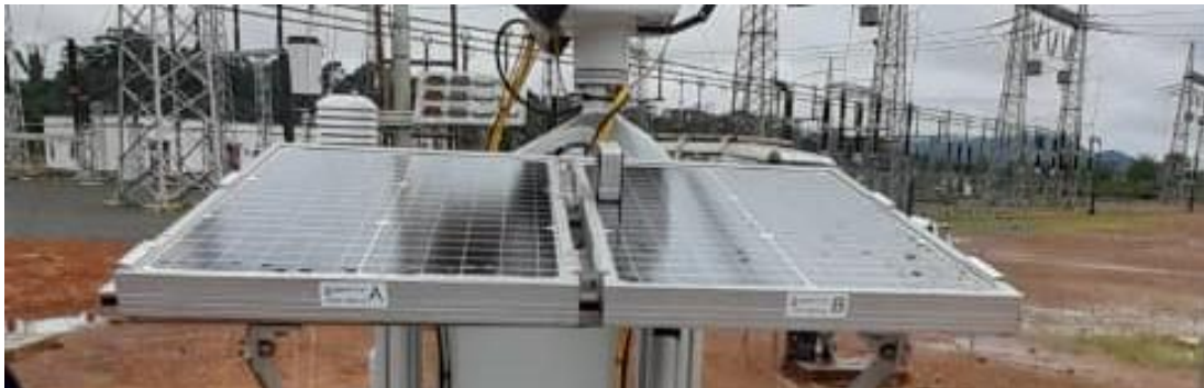
Figure 85: Assemblage de la structure PV-S + modules / Assembly of PV-S structure + modules.
