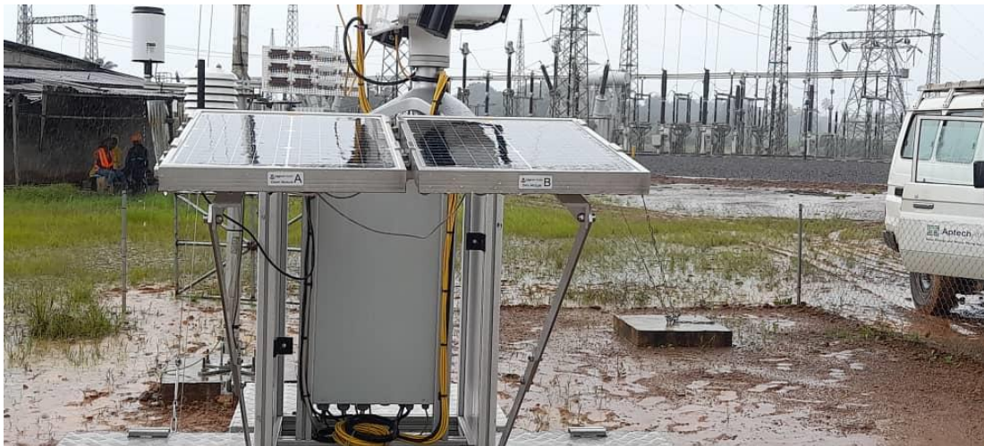
Figure 85: Assemblage de la structure PV-S + modules / Assembly of PV-S structure + modules.
