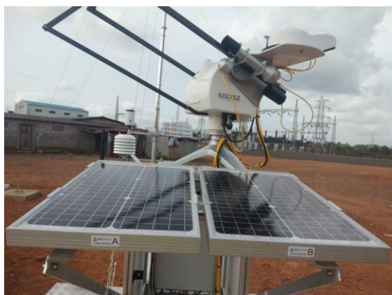
Figure 67: Assemblage de la structure PV-S + modules / Assembly of PV-S structure + modules.
