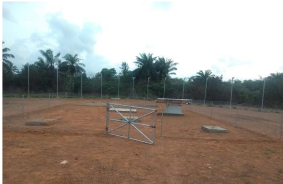
Figure 44: Clôture et fondation / Fence and foundations.
