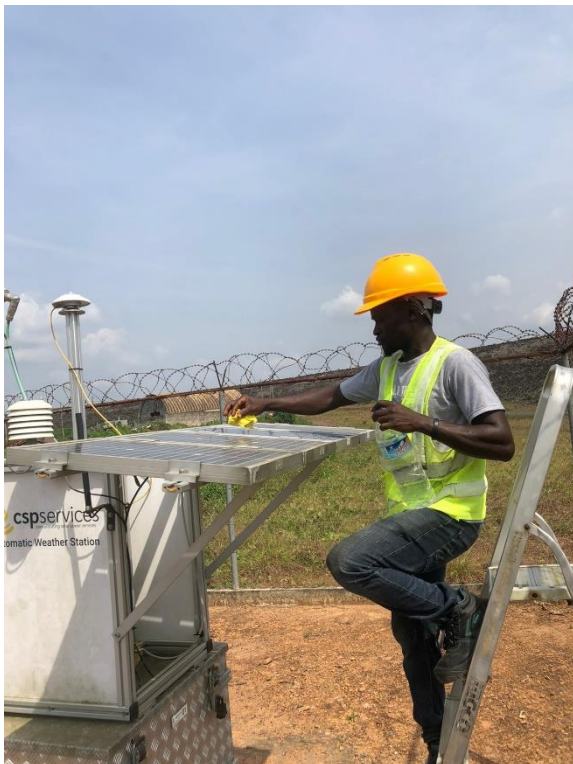
Figure 133: PV modules cleaning
