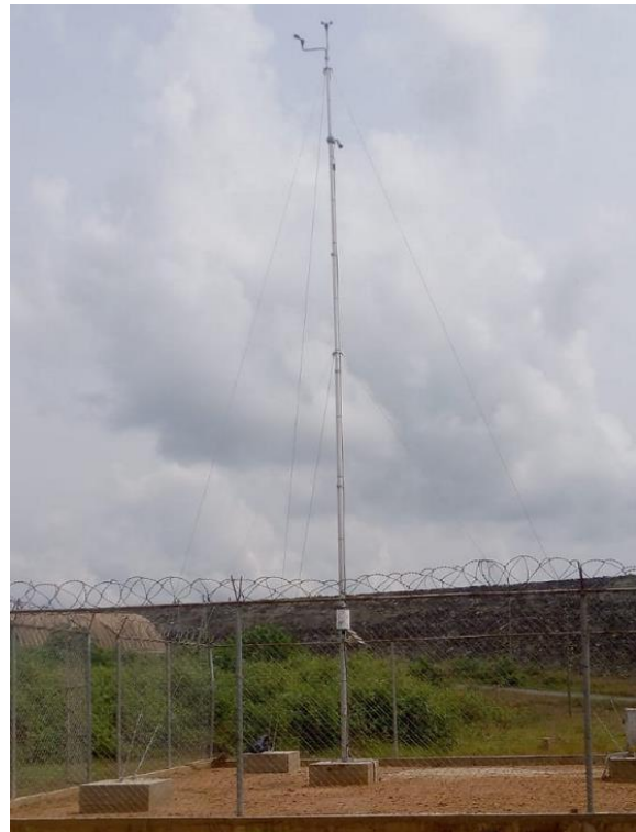
Figure 77: Wind mast with foundations and guying ropes
