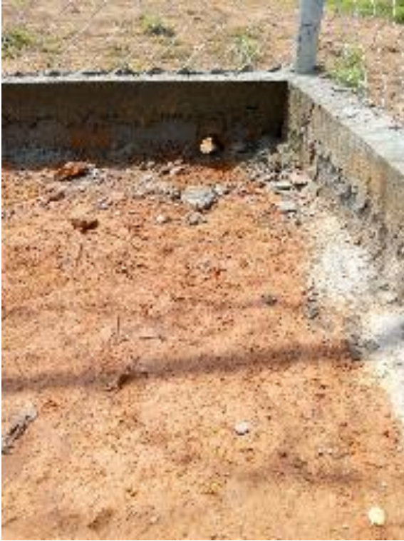
Figure 45 - Water holes in foundations to prevent flooding (1).
