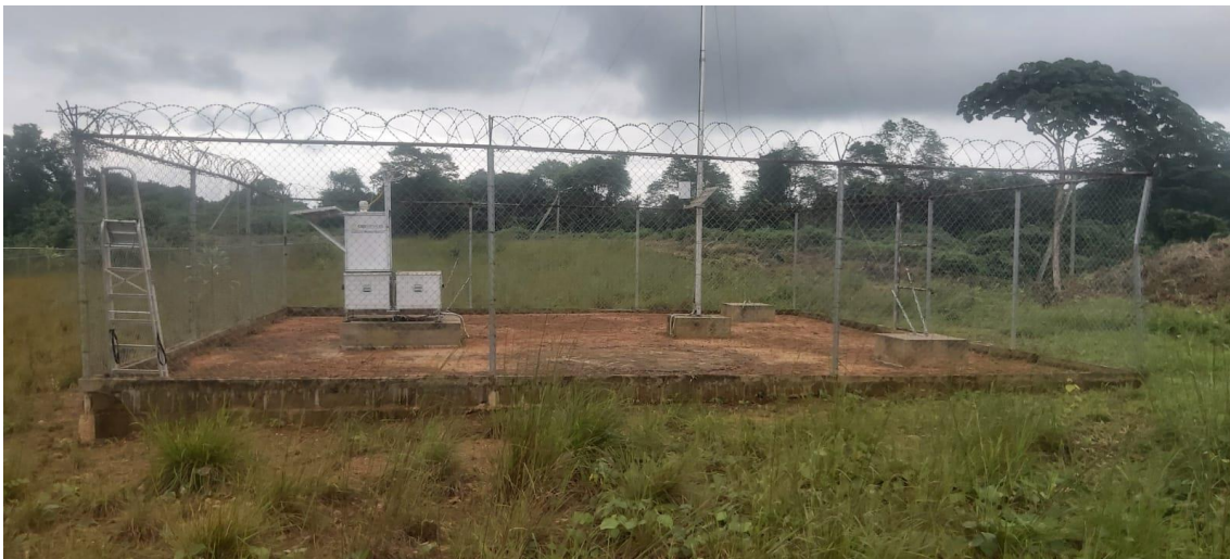
Figure 114: Site with completed station as seen from east
