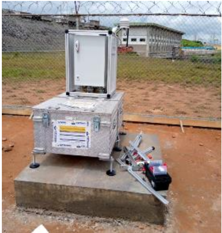
Figure 50 - Mounting of weather station structure
