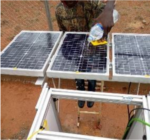
Figure 69 - PV modules cleaning.
