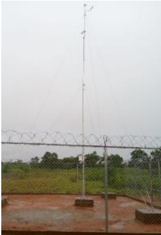
Figure 49 - Wind mast erected; wind direction sensor cantilever orientated to North
