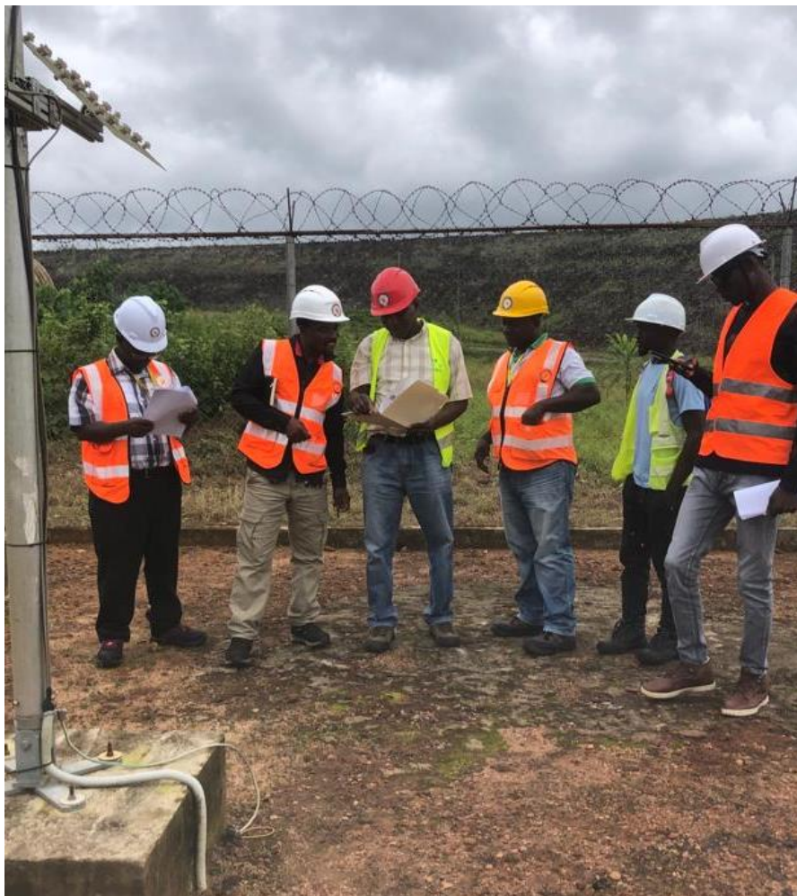
Figure 138: Station handover visit
