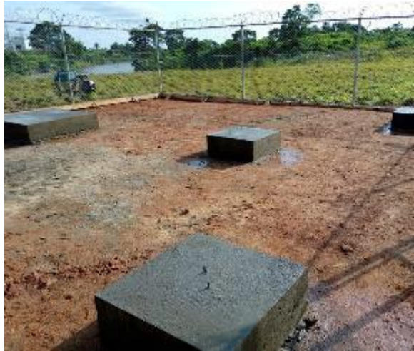
Figure 42 - Station and wind mast foundations
