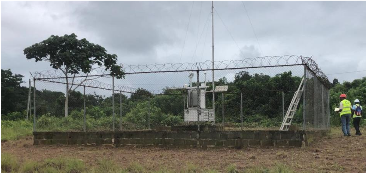
Figure 137: Station handover visit – view from south
