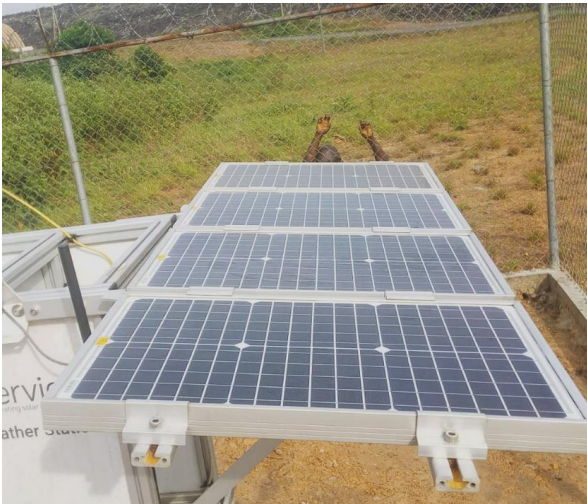
Figure 90: PV supply and soiling modules after cleaning
