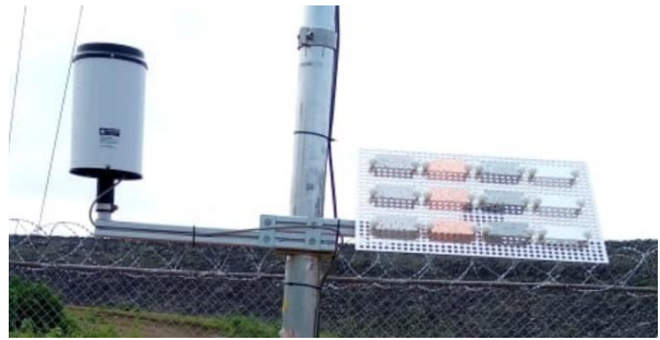
Figure 58 - Rain sensor and corrosion sampler
