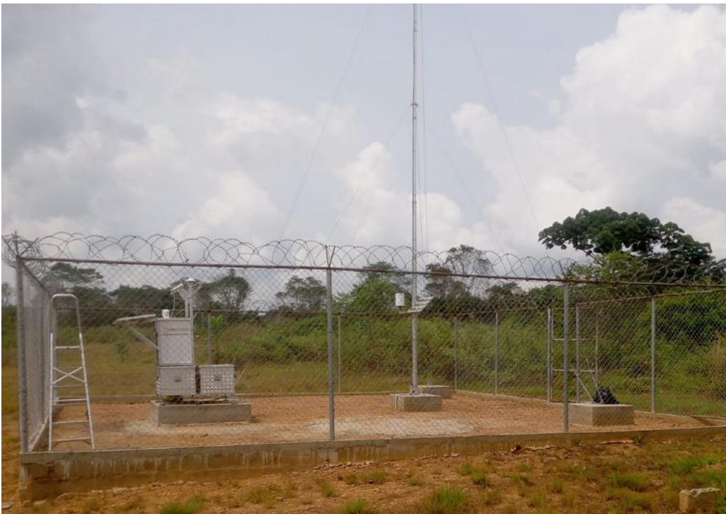
Figure 95: Site with complete station as seen from east
