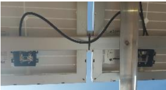
Figure 67 - PV-S modules connections
