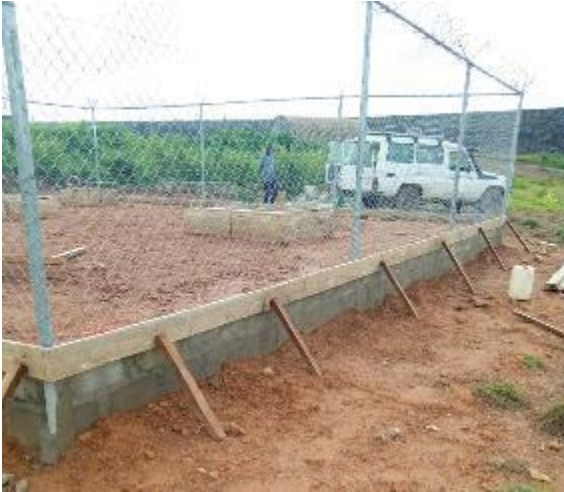
Figure 41 - Fence and foundation
