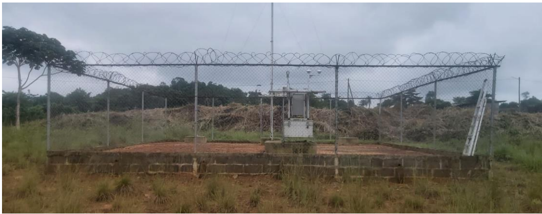
Figure 113: Site with completed station as seen from south
