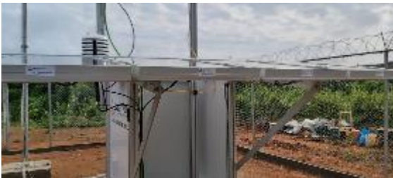
Figure 65 - Assembly of PV-S structure + modules
