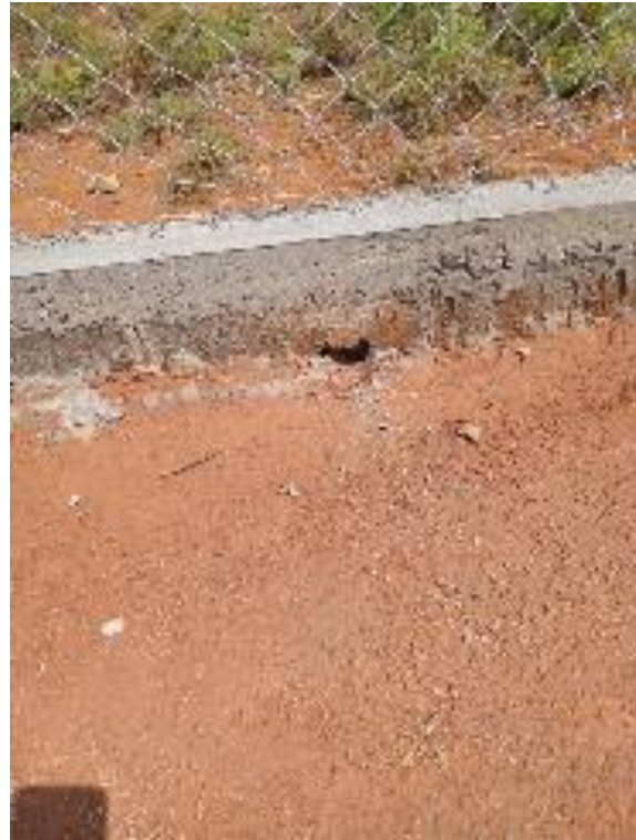
Figure 46 - Water holes in foundations to prevent flooding (2).
