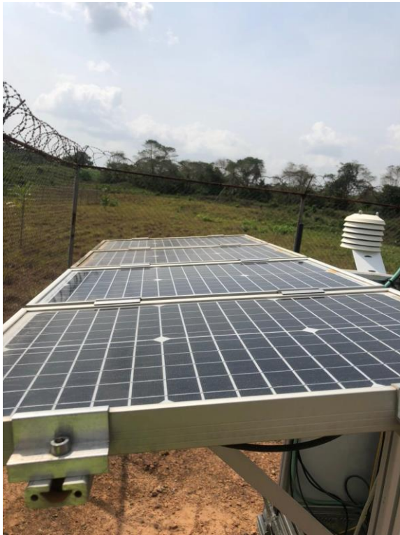
Figure 131: PV supply and soiling modules after cleaning
