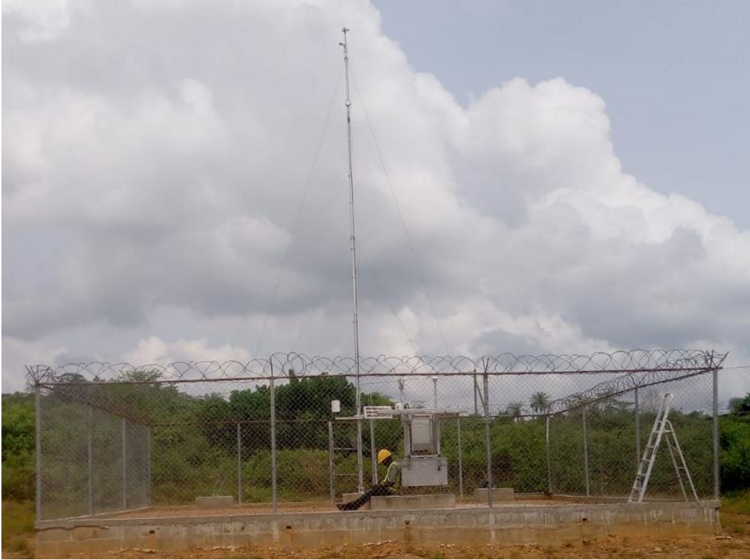
Figure 94: Site with complete station as seen from south
