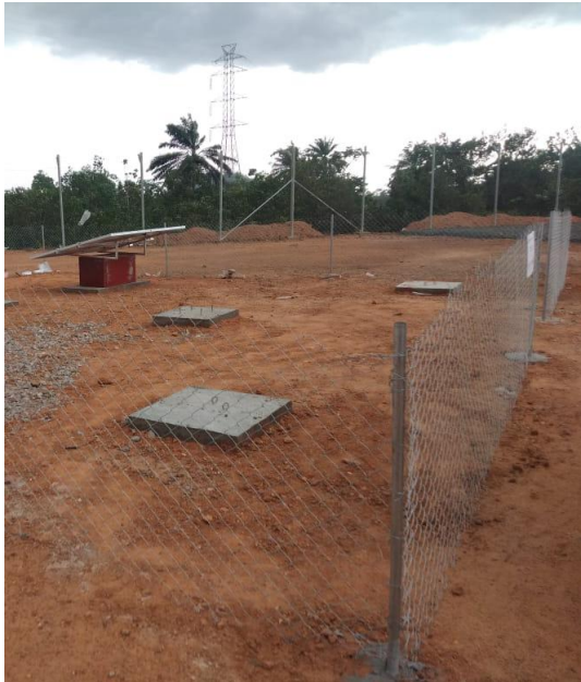
Figure 9: Clôture et fondation / Fence and foundations
