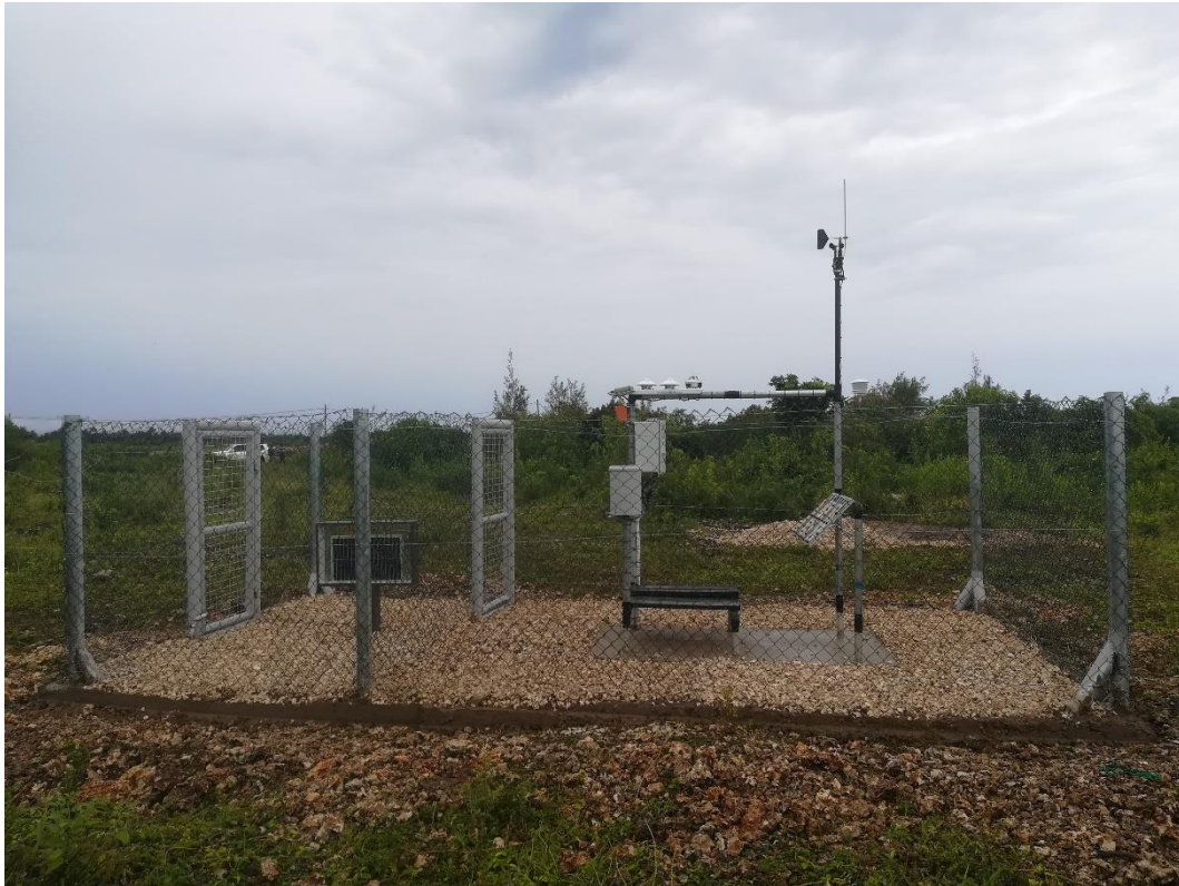
Figure 39: 270 Degrees (From West)
