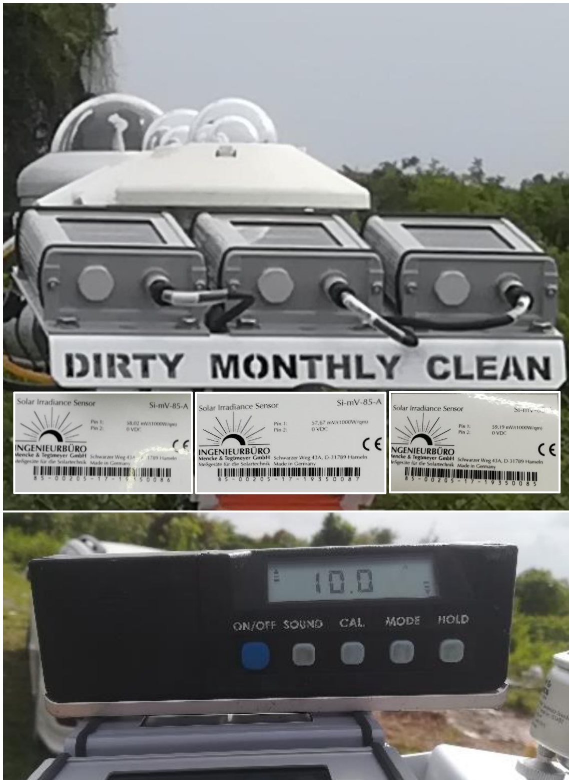
Figure 15: Reference Cells at 10° North
